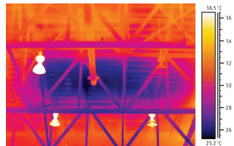
Figure 1. Thermogram during the morning from under a standing-seam metal roof, looking up at the underside of the deck. The sun has warmed up the dry areas of the roof, which appear red and orange. A wet section, not yet as warm as the dry areas, appears purple.
