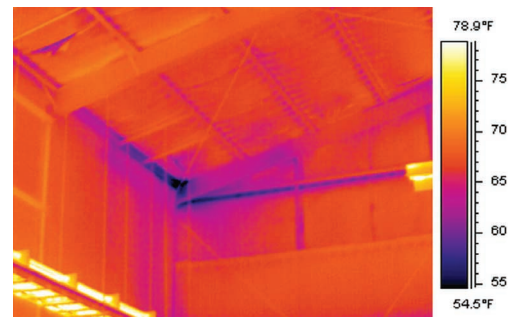
Figure 2. Thermogram of a leaky corner of a large electrical utility building, looking up at the underside of its standing-seam metal roof. The infrared emissivity of the wet materials is 0.98, compared with the emissivity of the metal roof itself, which is only about 0.01. Water has soaked the building walls as well as the underlying roof substrate.
